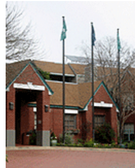
Habitat Suites Hotel installed a PV system in 2005.
