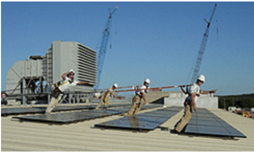
Meridian Energy Systems' crew installing the photovoltaic system at Sand Hill.
