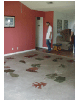
Volunteers have begun painting the concrete floor.
