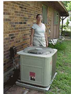
AYRW is proud of their new, high SEER HVAC system.
