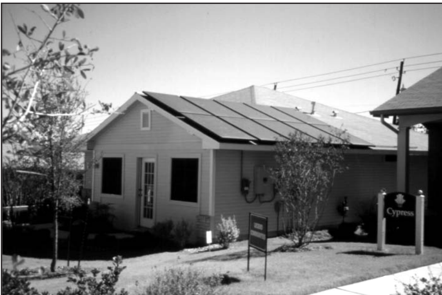
Retrofitted residential PV system The solar panels on the roof produce electricity that travels through wires to the distribution panel on the side of the home.
