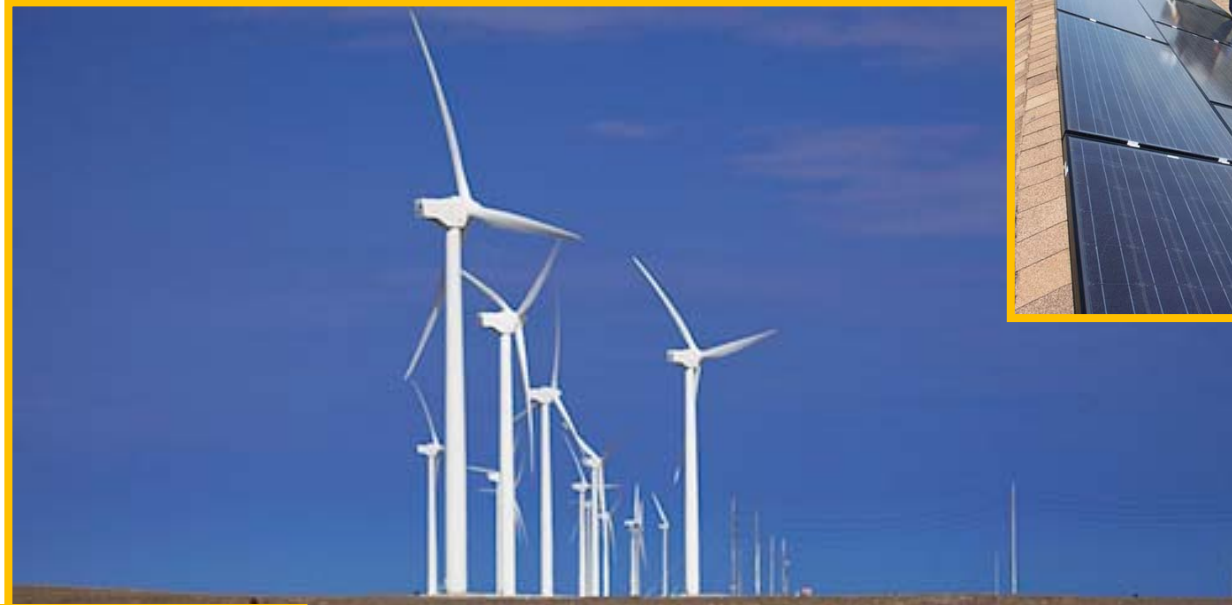
Wind Generation - Penascal Wind Farm, Texas, USA
